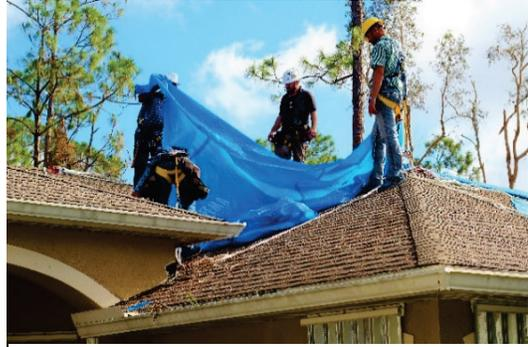
*Roofing contractors install FEMA supplied blue tarp sheets onto a Naples, Florida home in order to provide a temporary solution for residence housing shelter and prevent further damage after Hurricane Irma.*
